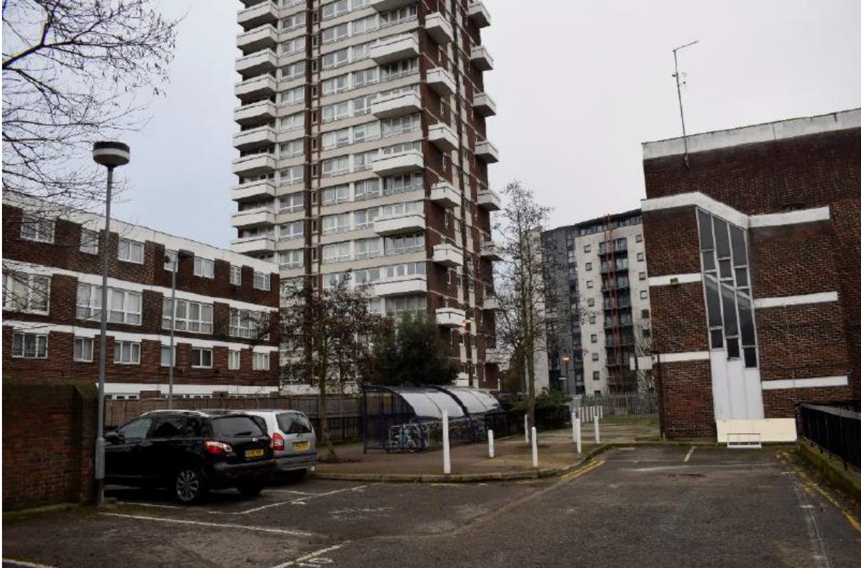
Photograph looking east, into the site, showing the 3 existing building and the western car park
